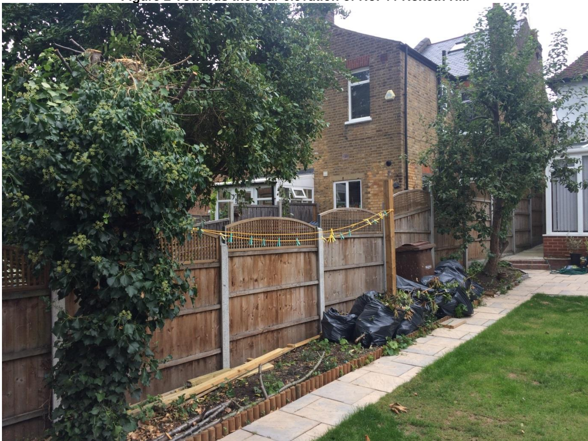
Figure 3 Towards the rear elevation of No. 40 Roxeth Hill
